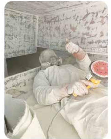
January 24, 2024: Sanding gelcoat
