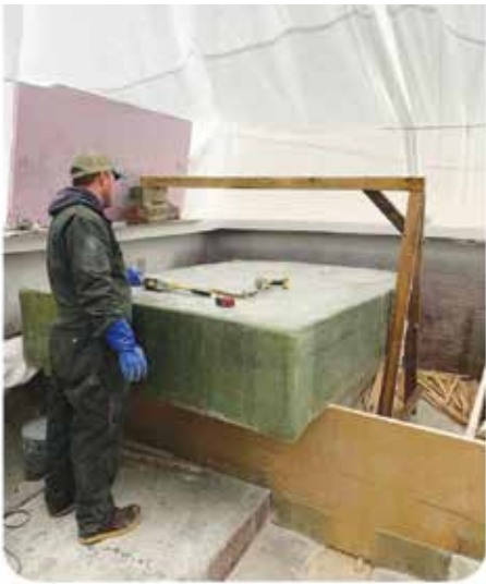
January 22, 2023: Setting fuel tank in place
