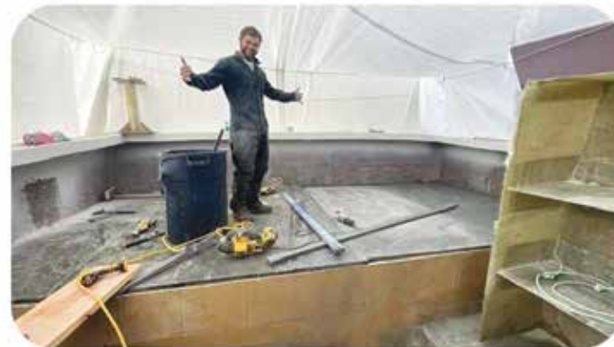
February 7, 2023: Got the first bit of deck down; portside fuel tank to the right
